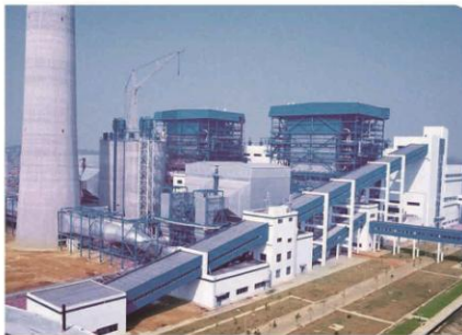
电厂输送粉煤灰系统 Power station flyash conveying system
