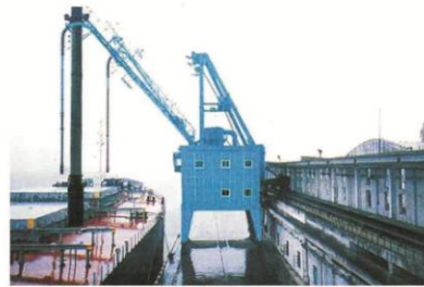
码头吸粮机 Suck grain machine in dock
